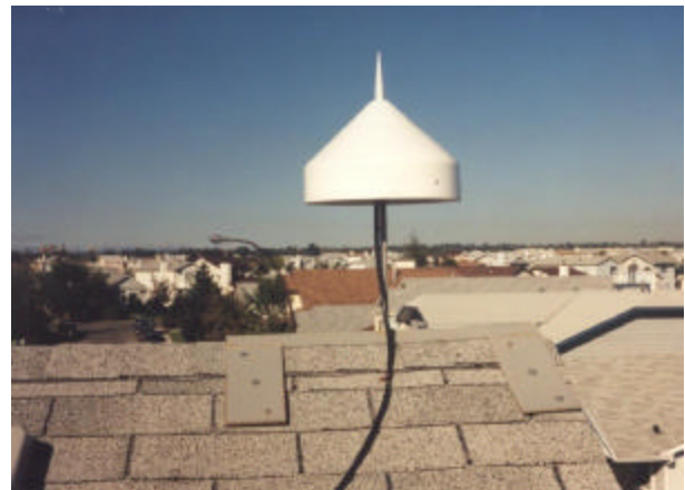
Figure 16: Choke ring antenna on a residential house
