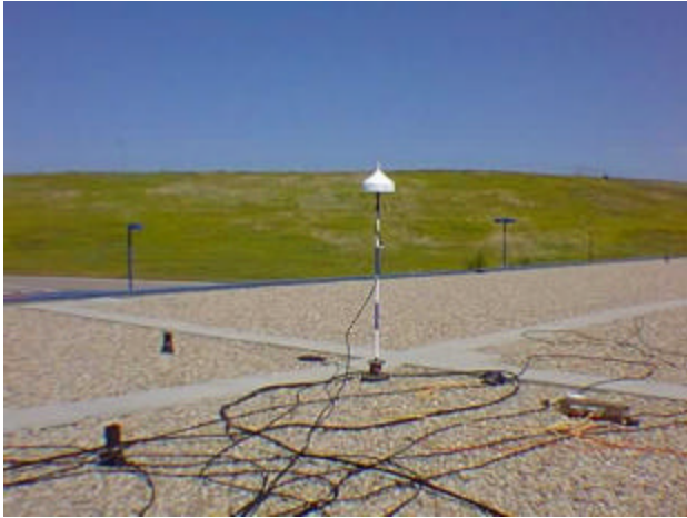
Figure 1: Roof of building
